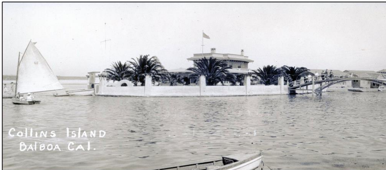
Figure 1: Circa 1930s photograph depicting the footbridge on the right (courtesy of the City of Newport Beach).
