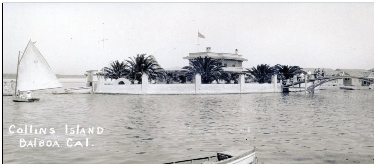
FIGURE 4: CIRCA 1930S PHOTOGRAPH DEPICTING THE FOOTBRIDGE ON THE RIGHT (COURTESY OF THE CITY OF NEWPORT BEACH)
