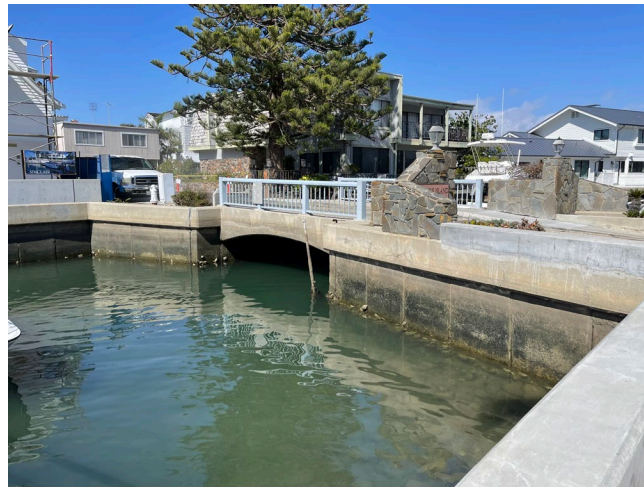
View looking at side view of existing bridge, seawalls, and infrastructure.
